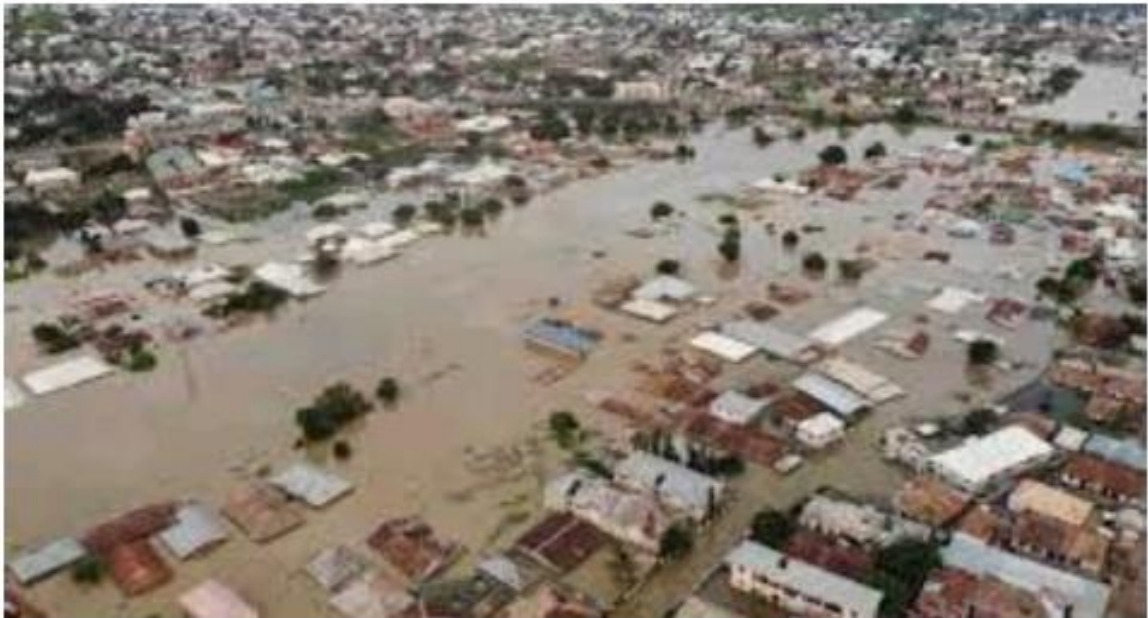
Plate 1: Aerial Photo Showing the Impact of the 2022 Flash Flood on a Section of Yenagoa
