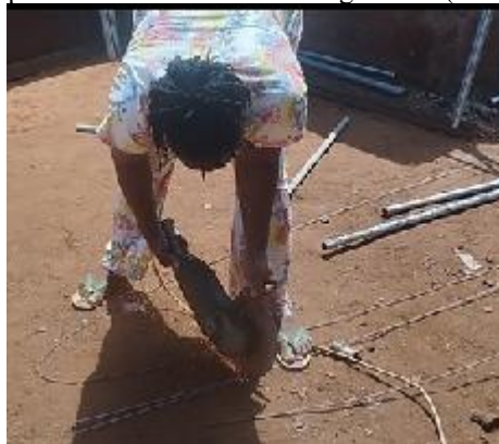
Plate 4: using power grinder to cut the rods for armature. Photo source: Osegbo C.O (2024)
