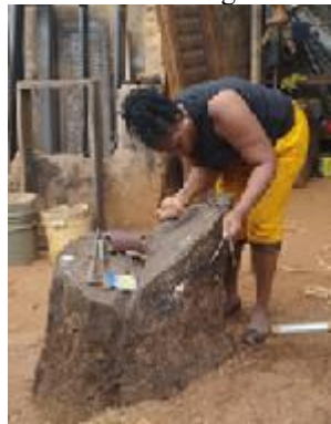
Plate 9: bending the rods to shape. Photo source: Osegbo C.O (2024)
