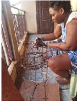
Plate 12: winding round the mature with binding wire. Photo source: Osegbo C.O (2024)
