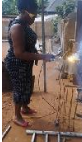
Plate 5: welding the pieces of rods to form the armature. Photo source: Osegbo C.O (2024)
