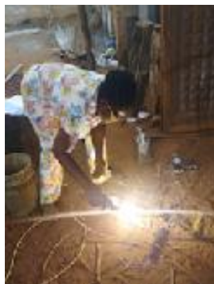
Plate 10: welding the pieces of rods to form the armature. Photo source: Osegbo C.O (2024)
